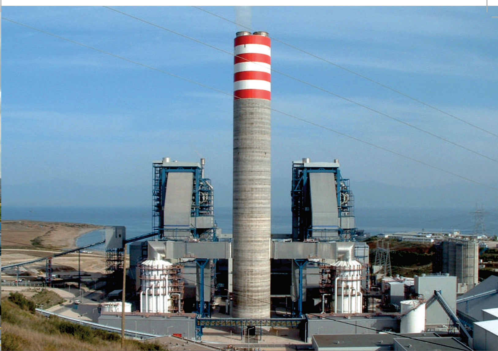
Sugozy Thermal Power Plant, Adana, Turkey
