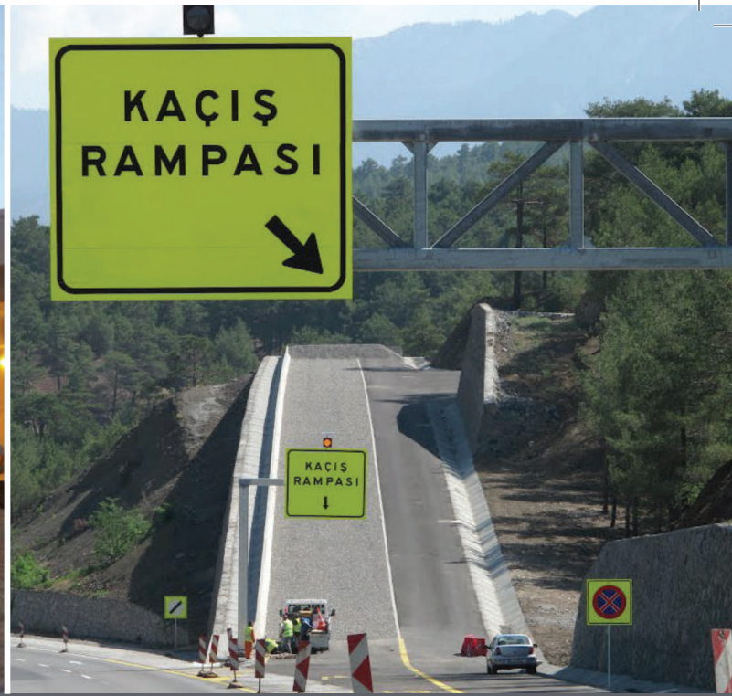
Ankara - Pozanti Motorway, Turkey
