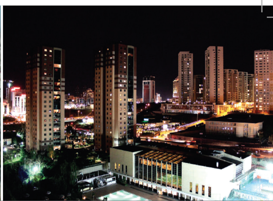
Ataşehir Satellite City Project, İstanbul, Turkey
