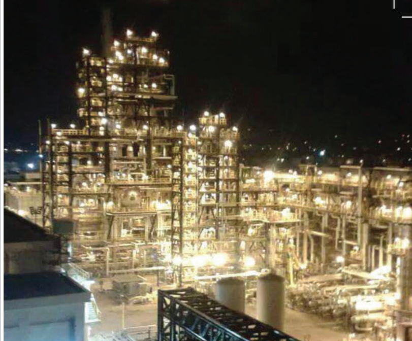
Tengizchevroil SGP Second Generation Project Refinery, Atyrau Kazakhstan
