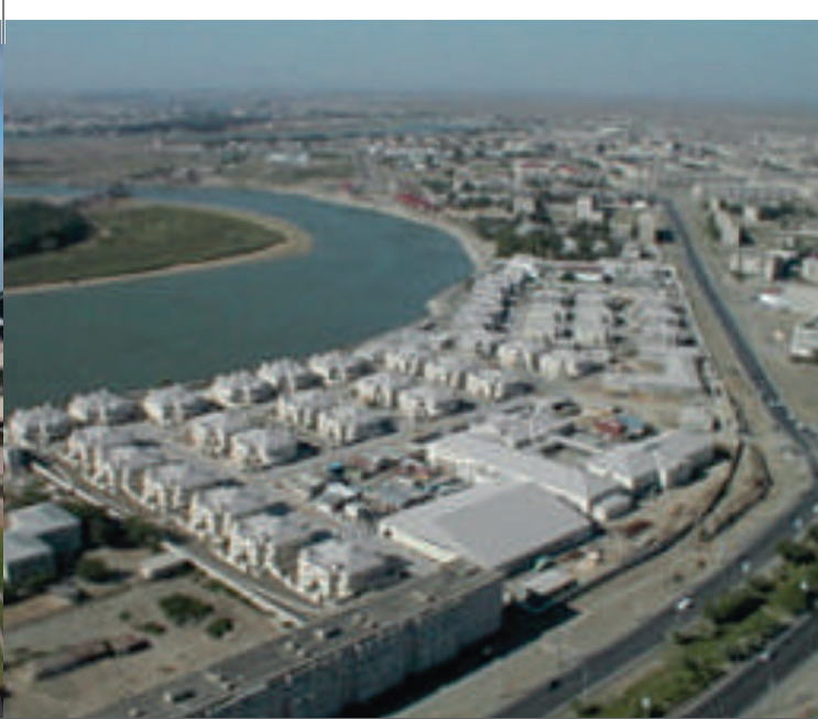
TCO Housing Project, Atryu, Kazakhstan
