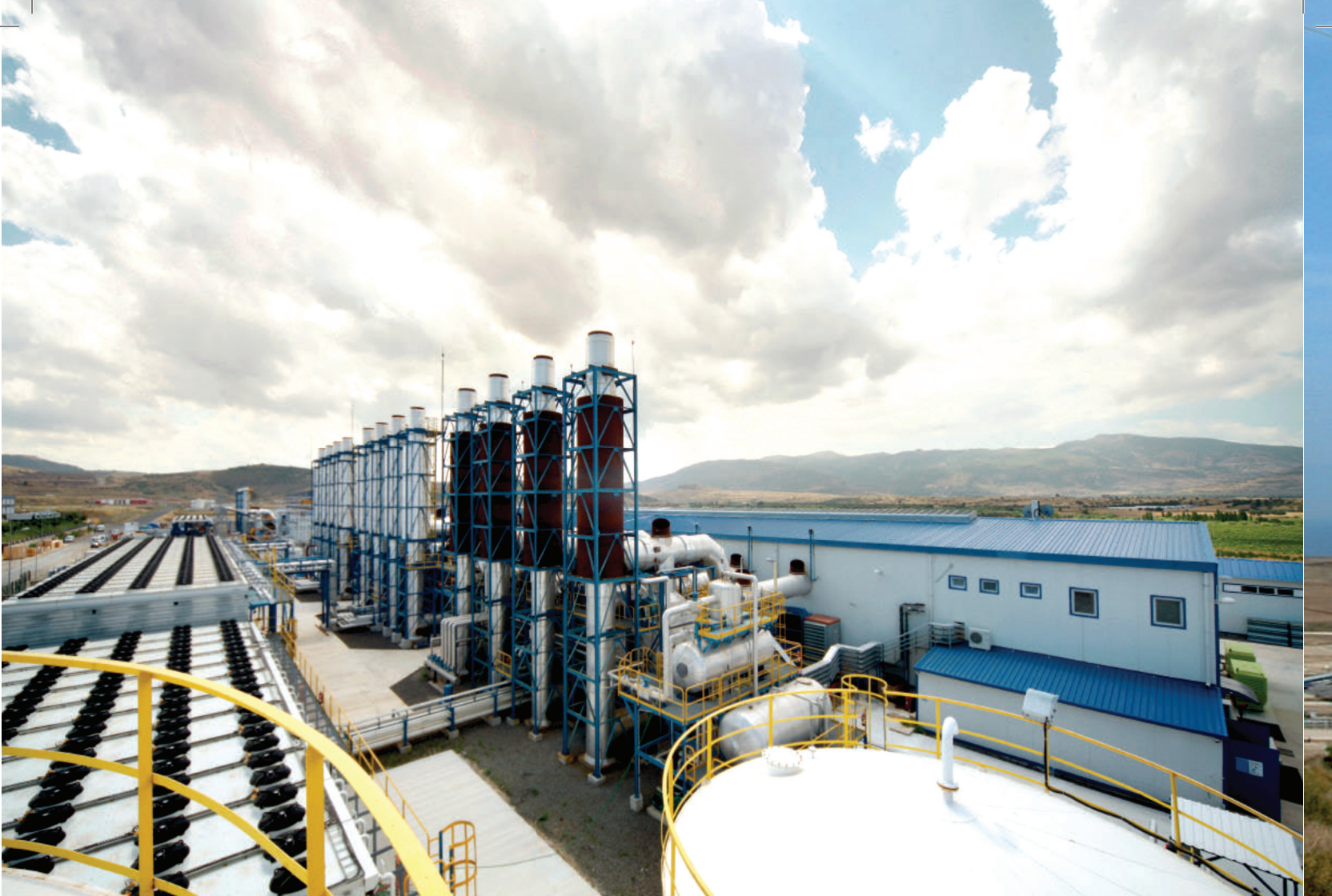
İzmir Aliaga Combined Cycle Gas Plant, Turkey
